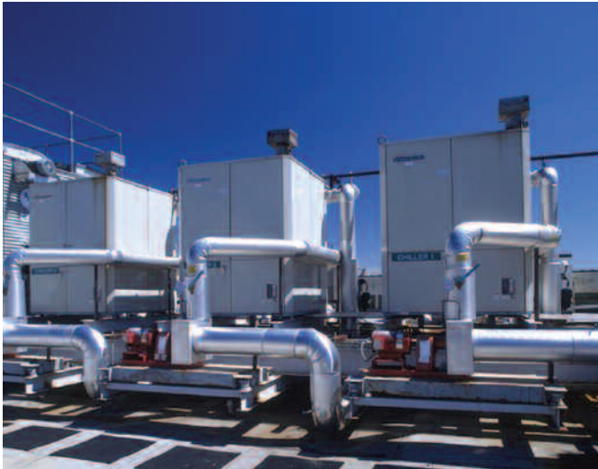
Trigeneration uses waste heat to drive absorption chillers (Yazaki Energy Systems)
