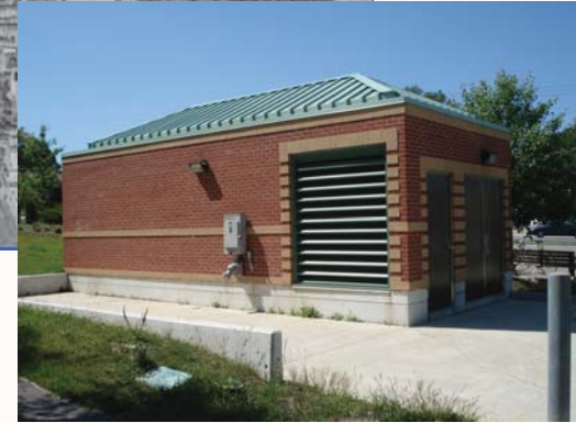
Emergency exit building on Bessarion Rd. Sheppard Subway
